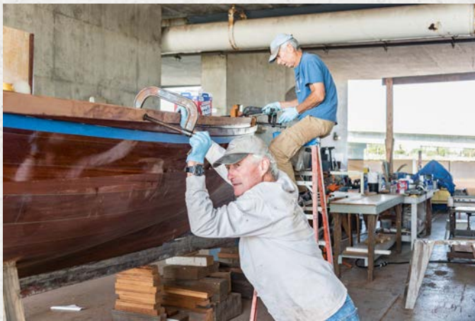
Volunteer John Kessler uses clamps to help bend the new ribs to the frame.
